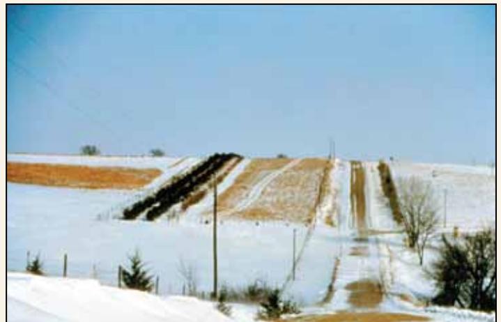
Living snow fences can be an effective way to control blowing and drifting snow, reduce snow removal costs and accidents.
