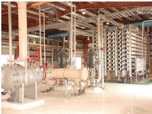
Brackish water desalination facility in Harlingen, Texas. The plant was built in 2007 and has a capacity of 2.25 million gallons per day. Source: North Cameron Regional Water Supply Corporation
