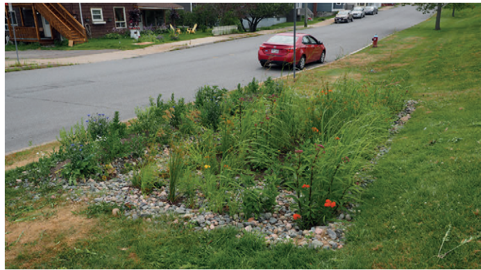
◀ Figure 18: In 2019, ACAP Saint John installed a rain garden on Queen Square West as a pilot project for the City. Green infrastructure can include implementing rainfall capture systems, permeable pavement, green roofs, bioswales, and rain gardens (Photo: ACAP Saint John).
