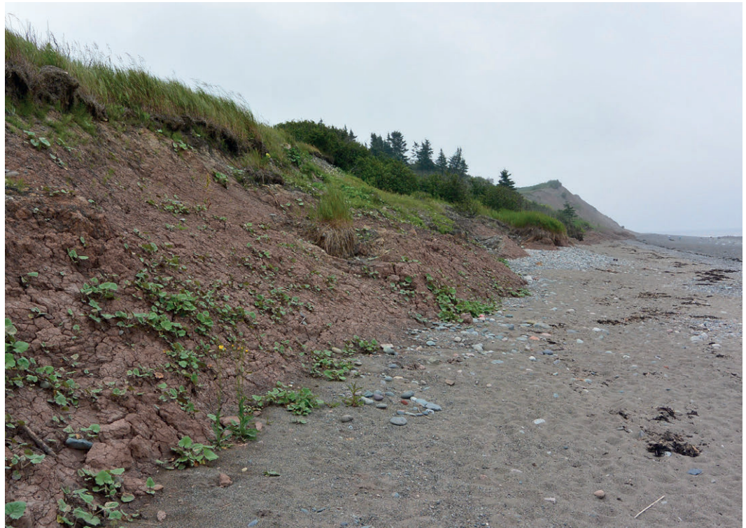
Figure 13: Shoreline erosion at Sand Cove Road in West Saint John (Photo: ACAP Saint John).
