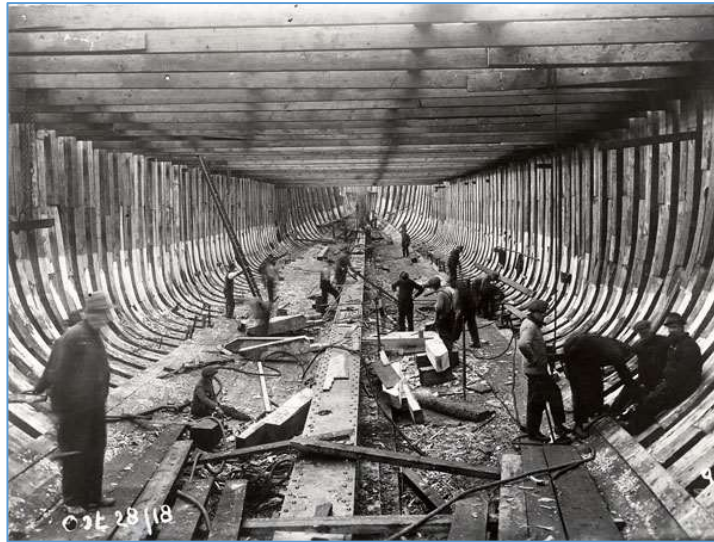
Figure 3. The photo shows builders at work in the interior of a boat. In the mid-19th century, shipbuilding was going full steam in New Brunswick. Each ship was built to its own specifications, depending on its intended use: hauling large cargos over the seas, speeding across the Atlantic, or carrying passengers. (Photo credit: Provincial archives of New Brunswick).
