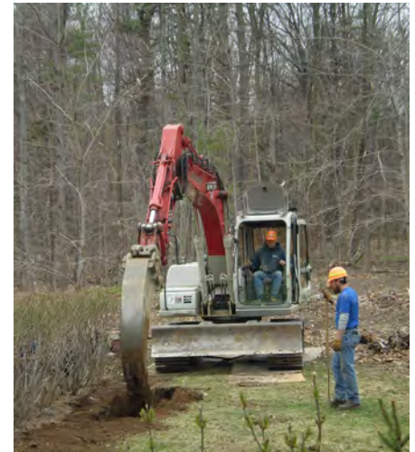
Trenching to break grafted roots
