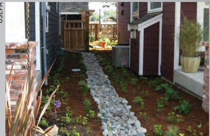
Roof downspouts direct runoff water to rock swales between homes.
