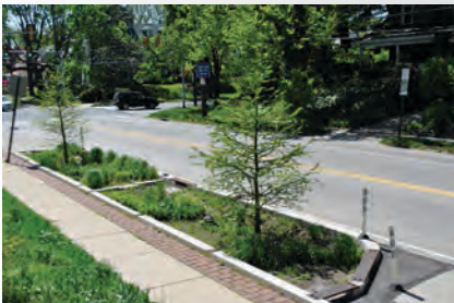
This stormwater curb bump-out intercepts stormwater runoff flowing down the street.
