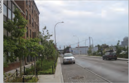
A permeable interlocking concrete paver parking lane is adjacent to a sidewalk planter.
