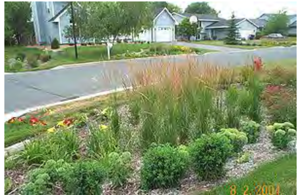
Photo illustrating a completed rain garden.
