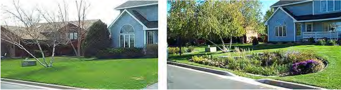
Photos illustrating a private residence before and after installation of a rain garden. Notice the curb cut from the street into the rain garden.
