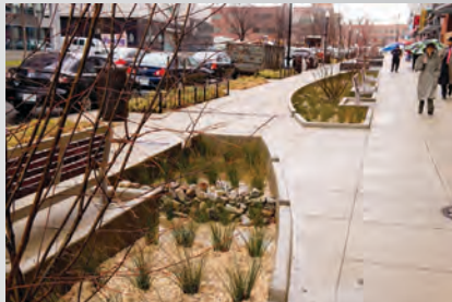
Runoff flows into stormwater planters installed in the sidewalk adjacent to benches.
