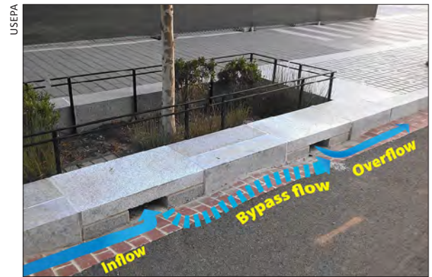
Figure 7. Bypass and overflow system. Runoff enters a planter box through a curb cut and collects until the practice's storage capacity is reached; additional water will either overflow through the second curb cut or will bypass the practice.
