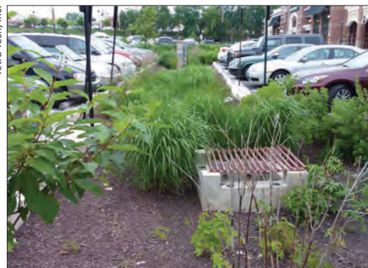
Figure 1. A parking lot bioretention area near Frederick, Maryland, is equipped with an overflow drain.
