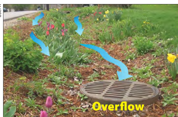
Figure 5. Overflow drain. Runoff water flows into this roadside bioretention channel, which is equipped with an overflow drain to prevent street flooding during high volume storm events.
