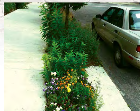
Stormwater planters in Philadelphia capture and filter stormwater runoff from an adjacent roadway.
