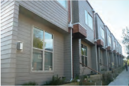
Roof runoff enters bioretention flow-through planters for treatment and short-term storage.
