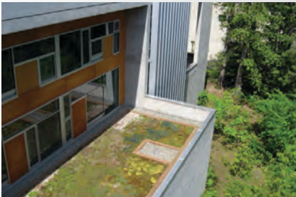
A building's green roof captures rainfall, thereby reducing local runoff.
