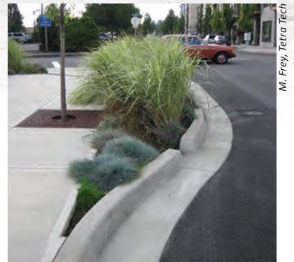
Curb bump-out creates narrower streets and captures runoff, Gresham, Oregon
