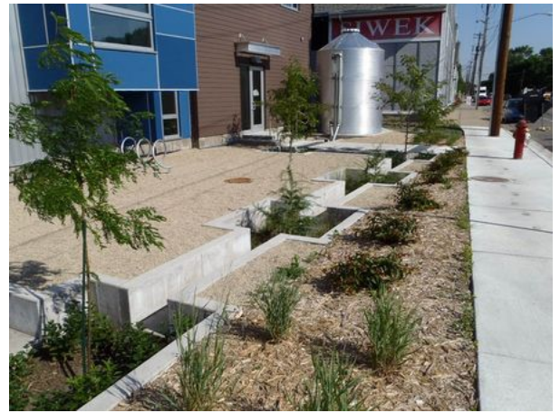
Cistern located at Mississippi Watershed Management Organization. Photo by MWMO Staff. To enlarge,click on image.
