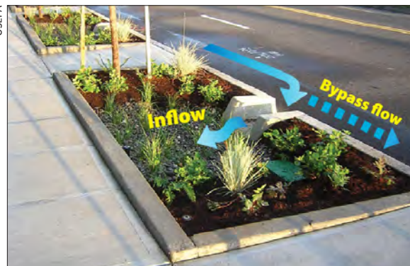
Figure 6. Bypass system. A curb cut allows street runoff to enter this sidewalk planter. If the planter fills completely, additional runoff water volume will be forced to bypass the practice and continue flowing down the road.
