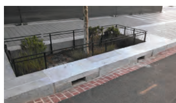
Stormwater runoff flows through roadside curb cuts into a sidewalk bioretention planter.
