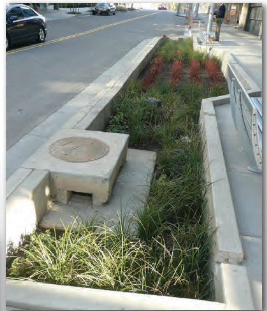
A stormwater planter tucked along the edge of the roadway captures and treats street runoff while also providing an aesthetically pleasing green element within the urban waterfront district.
