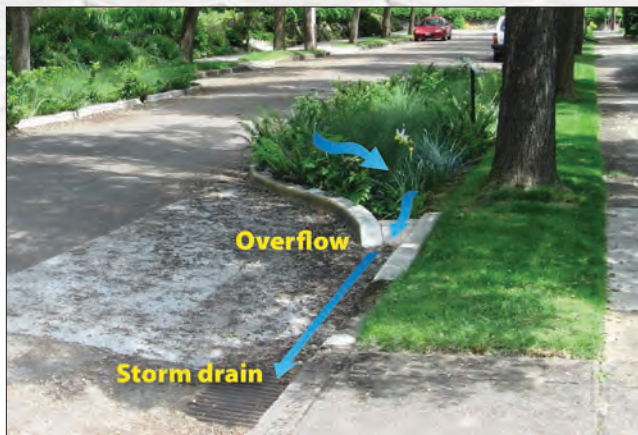
Figure 3. Street runoff enters the upper end of this bioretention area and fills the practice. The overflow volume exits through an opening on the lower end and drops into a storm drain.
