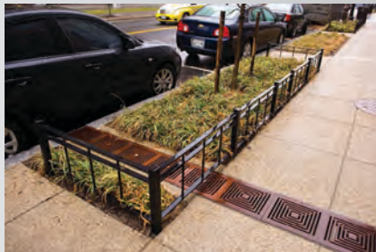
A bioretention cell receives stormwater runoff through a curb cut and surface grate.
