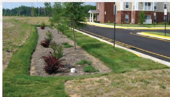
Stormwater infiltration trench, Stafford County, Virginia
