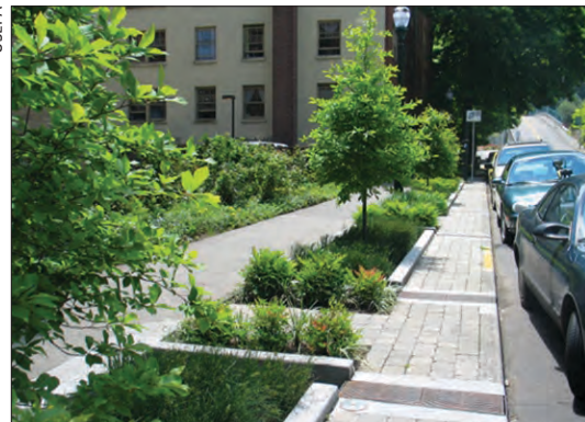
Figure 2. Stormwater planters treat runoff and can bypass flows that exceed their treatment capacity.
