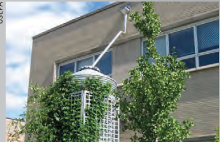
A cistern collects rooftop runoff, which is used to water landscape areas around the building.
