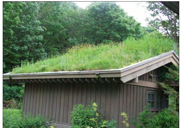
Figure 4. Green roofs provide many benefits, including their alternative roofing material.
