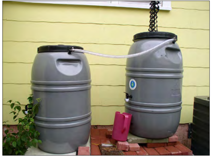
Figure 1. Two rain barrels can be linked so that, as one fills, any overflow goes into the other container. It is important to provide sturdy bases so that the barrels won't topple over.
