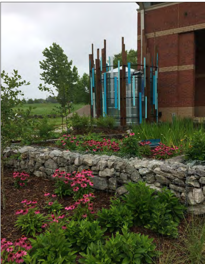
Figure 2. Rain gardens, such as the one at the Mississippi State University Landscape Architecture Facility, are designed to channel and filter excess rainwater.
